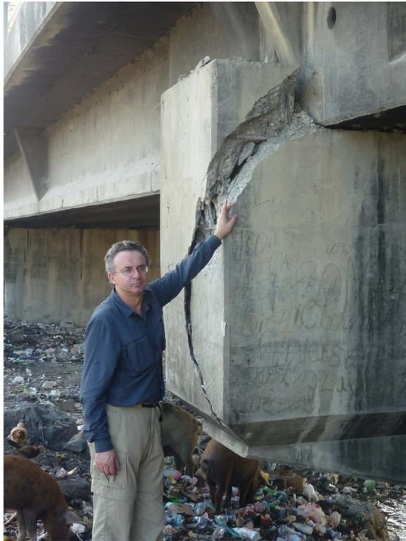
**Figure 9.** Damage to shear key at intermediate support.
