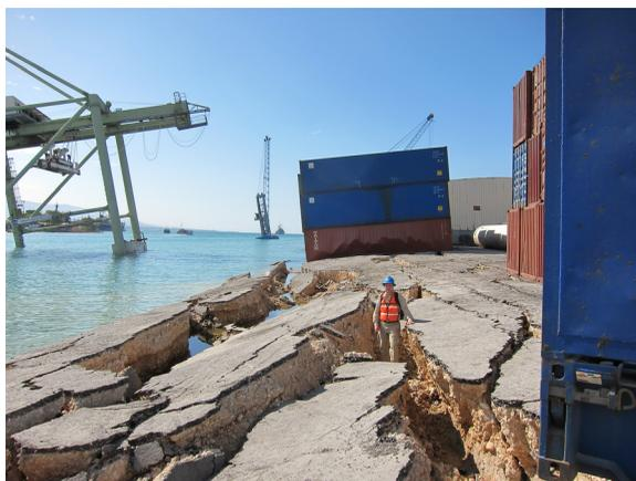
**Figure 4.** Liquefaction-induced lateral spreading leading to the collapse of the North Wharf at the Port de Port-au-Prince.
