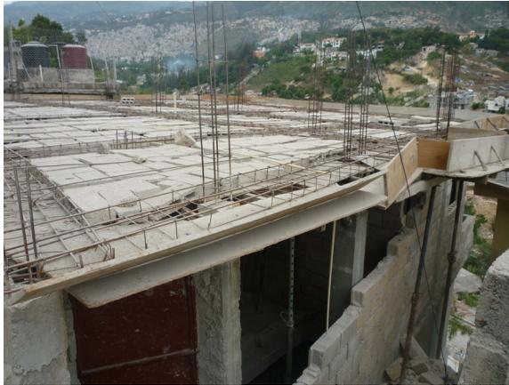
**Figure 5.** Residential concrete block slab construction.
