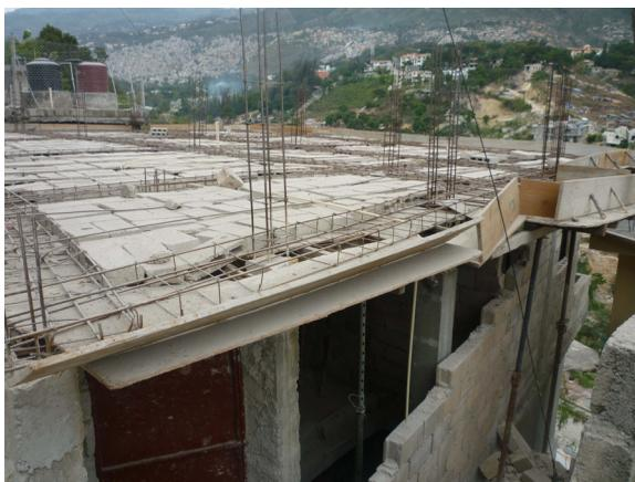
**Figure 5.** Residential concrete block slab construction.
