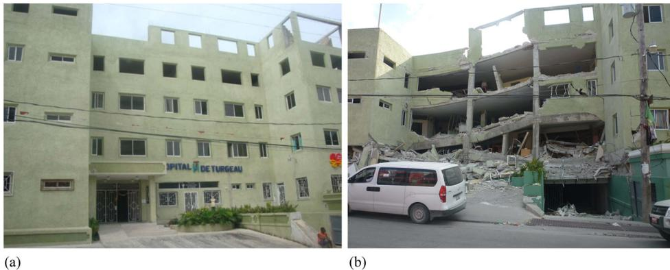
**Figure 6.** Turgeau hospital in downtown Port-au-Prince: (a) Before the earthquake (Simon Young CaribRM), and (b) collapsed structure after the earthquake.
