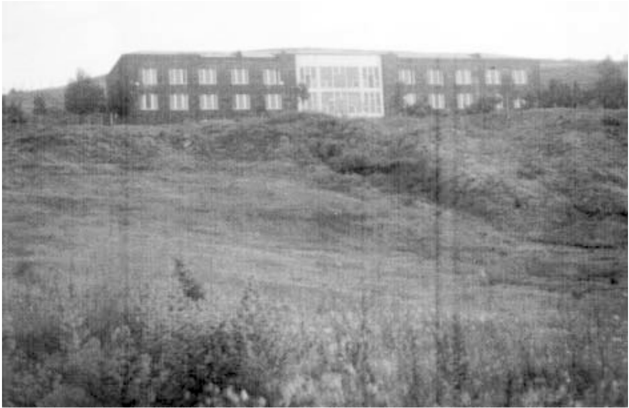
Figure 2-7. Two-story building at Garni Observatory.
