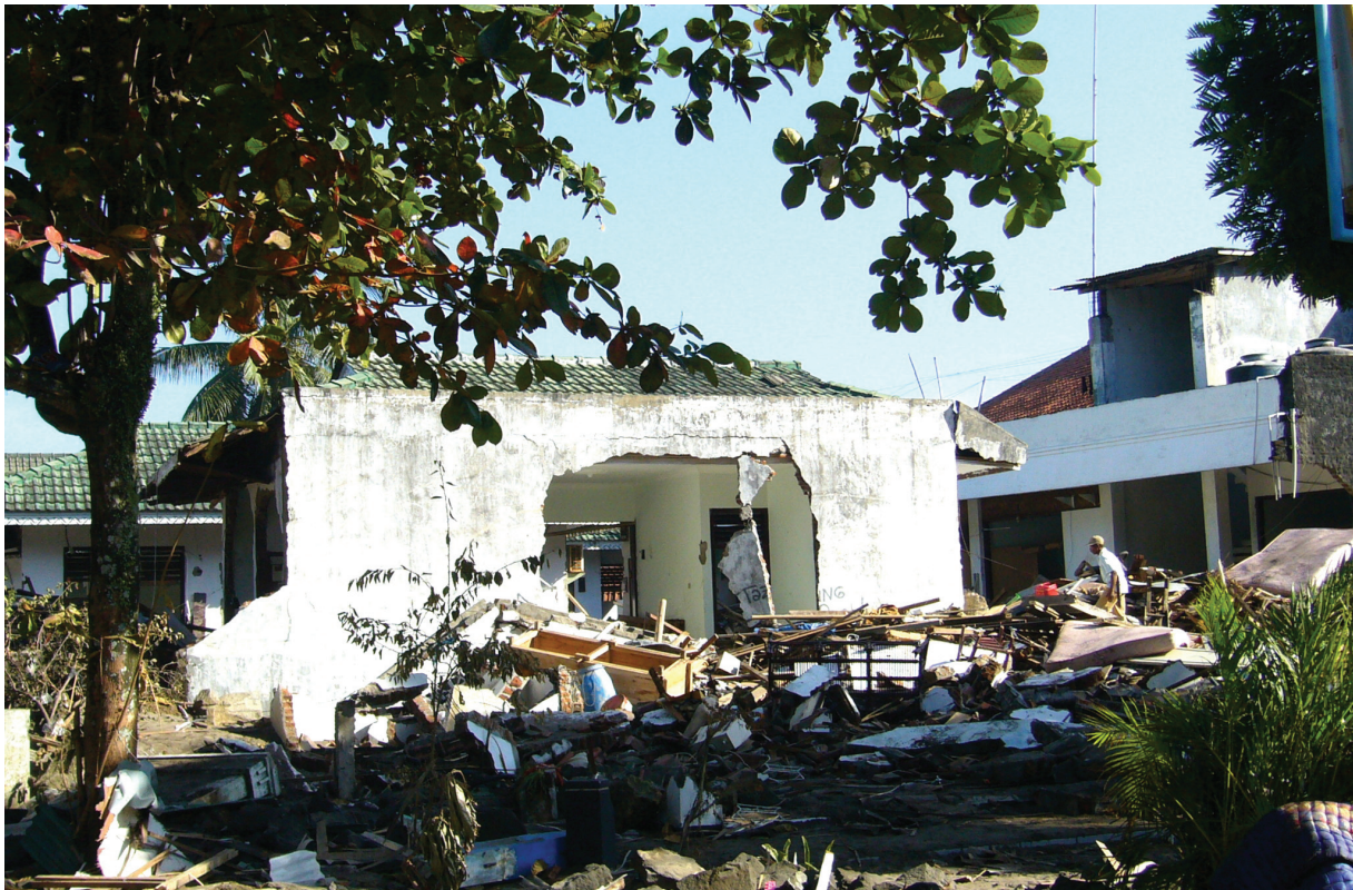
▲ Figure 4(A). Tsunami damage to unreinforced masonry buildings and debris in Pangandaran.
