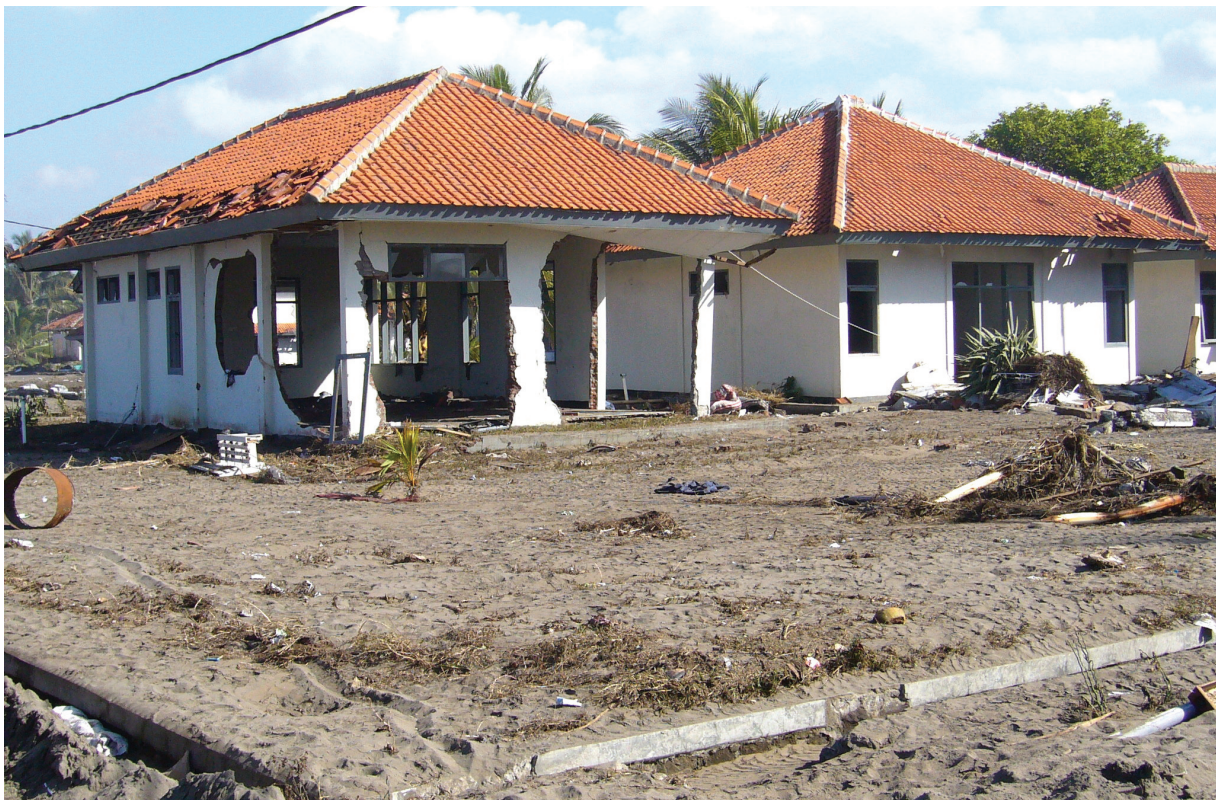
▲ Figure 4(B). Damage to buildings near Pangandaran. Note the damaged roof on the building on the left, which indicates the height of the tsunami.
