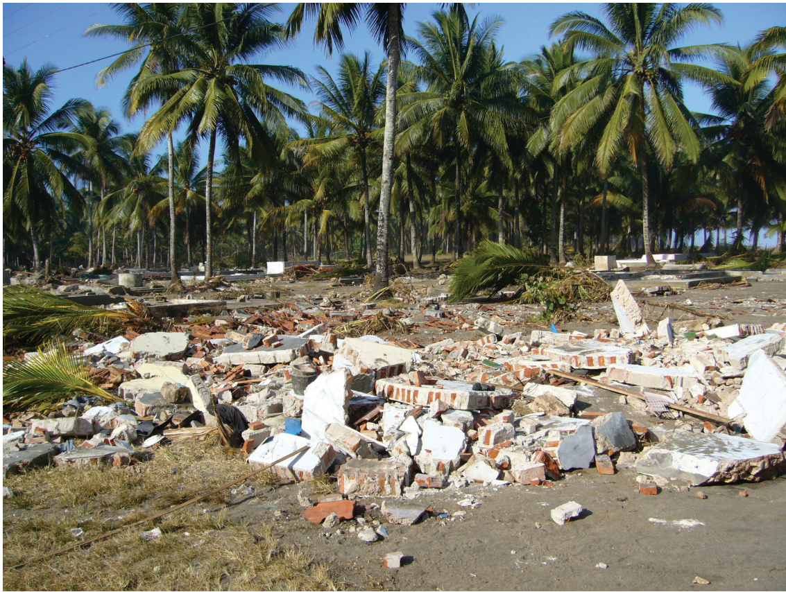
▲ Figure 5. Severe damage in Marsawah village, where no walls were left standing within about 150 m of the shore.
